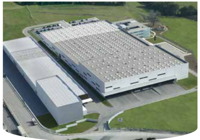
Research & Development and Manufacturing facility in Gijón (Spain)
